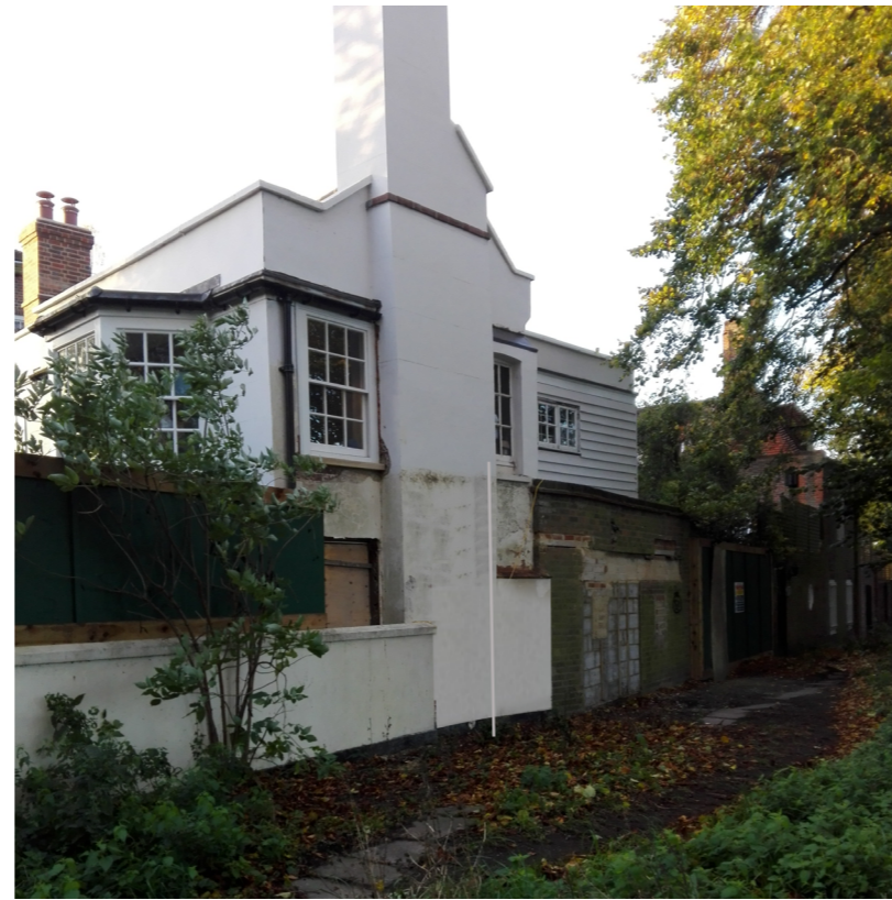
LOCATION A WITH POLE
