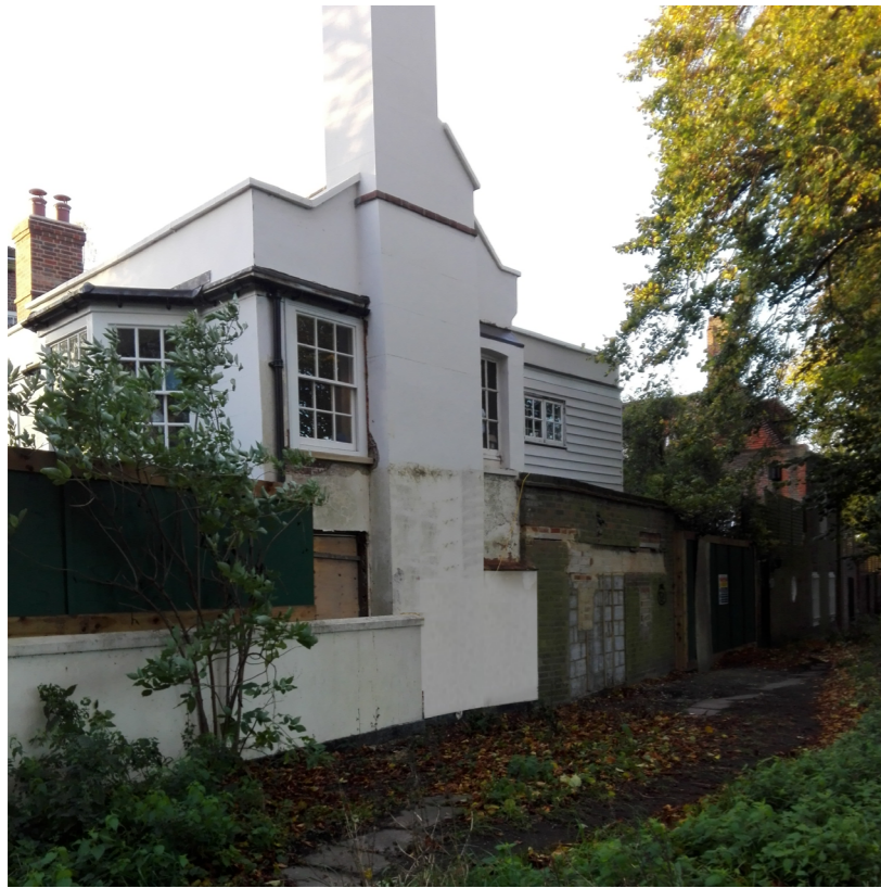
LOCATION A WITHOUT POLE
